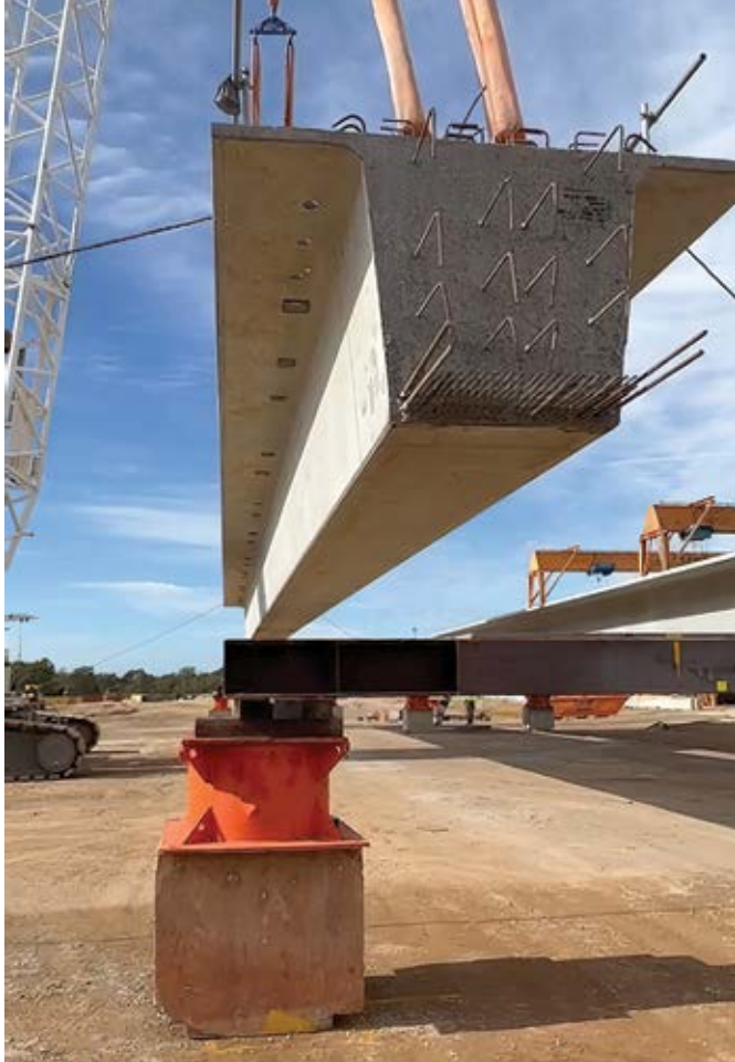
Project: Mitchell Freeway Extension Location: Perth, WA Master Precaster: PERMAcast
