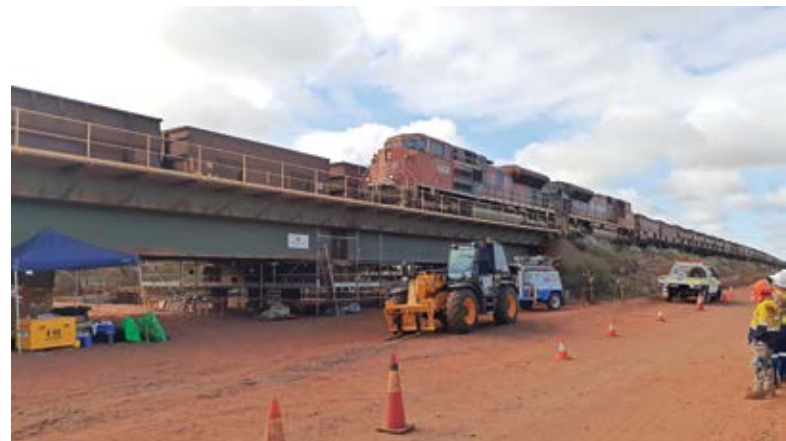
mageba supplied custom bearings for a multimillion-dollar, multi-stage rail project in the Pilbara region of Western Australia.
