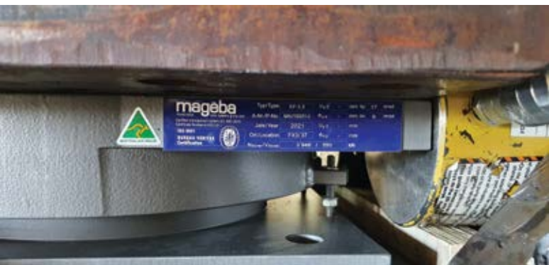
TOP: Installing one of the bearings along the Pilbara rail bridge. ABOVE: The bearings are load tested to ensure performance.
