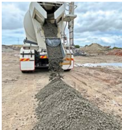
MasterSuna RCT 323 allows ready-mixed concrete producers to convert returned fresh concrete into a usable material suitable for use in a range of applications including road base and construction backfill quickly and efficiently, without the need for any additional specialist equipment.
