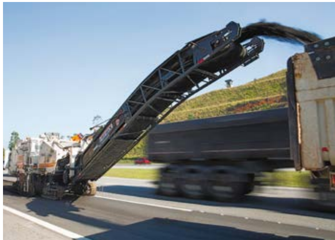
With a maximum milling depth of 320 mm, the Wirtgen cold milling machine W 1900 can remove entire pavements comprising the surface, binder and base in a single pass, saving time and ensuring high productivity.
